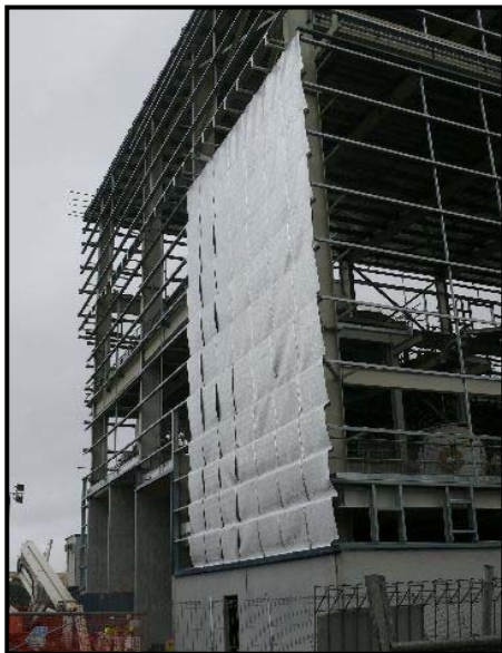
Application of "pyrotek" a noise control product.
